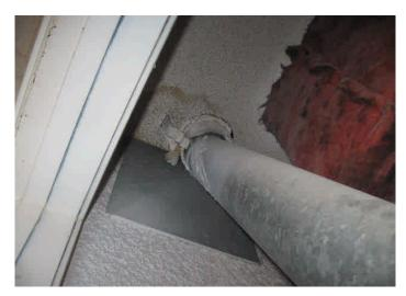
Ceiling stains noted around the furnace vent pipe at the ceiling were dry-recommend further investigation to insure that any leaking and moisture damage has been corrected.
