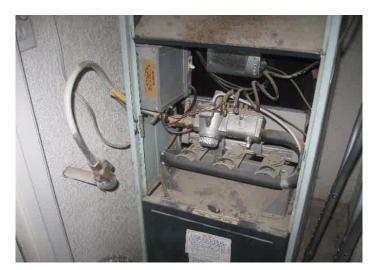
The gas feed line to the furnace is an old, rigid, aluminum type that is recommended to be replaced by an appropriate specialist with a currently approved stainless steel flex type.
