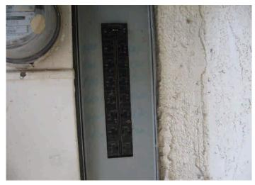
The interior-dead front cover on the electric panel has the screw missing that secures the cover, this should be replaced with a screw that is not pointed so that it will not as likely damage electrical wiring insulation if it comes in contact with wiring.
